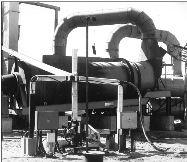
Impedance heating used to maintain temperature of 350 tons of asphalt.
